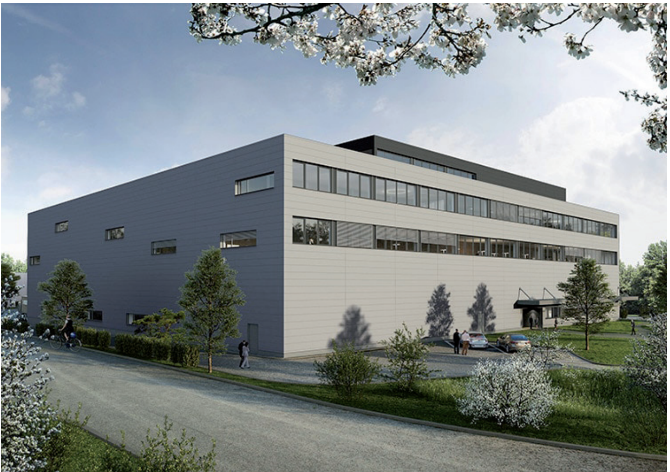
View of the new building in Oftringen
